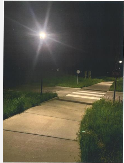
View from W.19th St., looking east, into the covered 6th Ave., overpass area.
