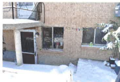
Exterior of apartments, stairs leading to garden level door (center), bathroom window (right), potted plants (far right).
